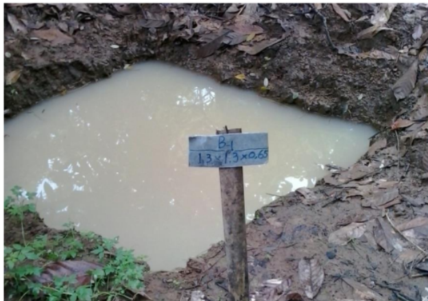
Figure 3. Building of zero run off.
